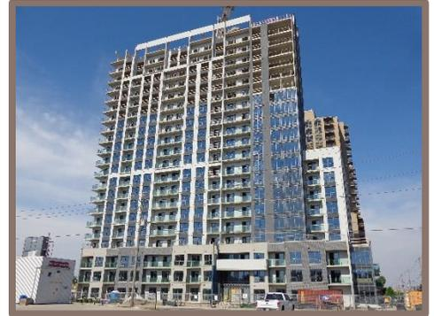
King and Lyle Apartments is a 21-storey total precast apartment building consisting of (298) one, two & three bedroom units ranging from 350 to 1400 square feet. The 3-storey podium effectively uses precast panels with brick and block form liners to create an approachable street scape. The Buildings facade steps back at the 3<sup>rd</sup> floor as well as the 10<sup>th</sup> floor.
