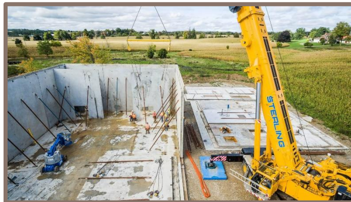
LIFTING PANELS The fully insulated panels provide and energy efficient envelope.
