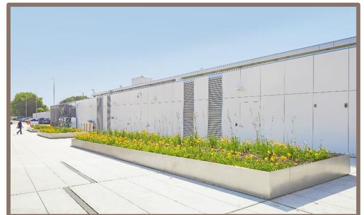
The building plays an integral role in supporting the station's daily operations as it houses the boilers for the platform snowmelt system, electrical and communications rooms and generator. Moreover, it encompasses a rear wall design spanning 3m tall and 450mm thick that functions as a retaining wall to resist train loading, enable future rail expansions and support the sloping green roof which is supported by a 350mm-thick concrete slab.
