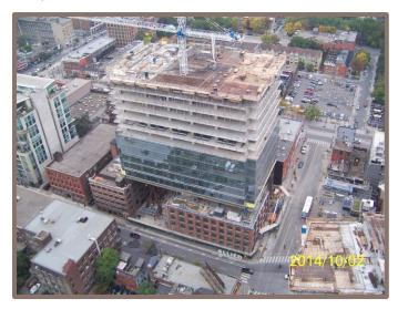
The 7th floor structural steel "table top" provides the base for the concrete tower. The table top is supported by 2 concrete elevator cores, one concrete stair core, new concrete floors and columns in a heritage 5 floor building (replacing the original wood structure) and 3 structural steel, concrete filled "delta frames".
