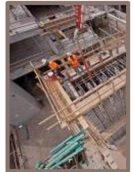
PCR Contractors used many of the CBM Maximizers during the construction over many seasons, from Mid-Range and High Range plasticizers to full Self Consolidated Concrete mixes on some of the exposed columns. In order to accelerate the schedule and reduce shoring requirements, the CBM First Up mix was used in most of the beams that supported the hollowcore flooring. Designed to give 75% within 2 or 3 days, PCR was able to strip the forming and didn't need to re-shore the structure.
