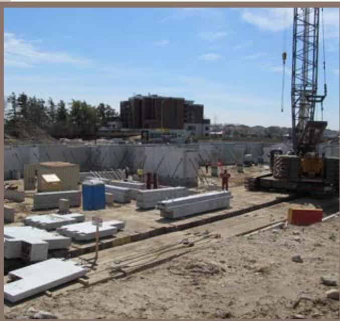
Precast concrete product's inherent fire resistance eliminated the need for a great deal of fire-proofing that would be required for other building materials, saving time and money and subsequent repairs. Precast also offers great sound control features, with the hollow core slab by itself receiving a STC rating of 50.
