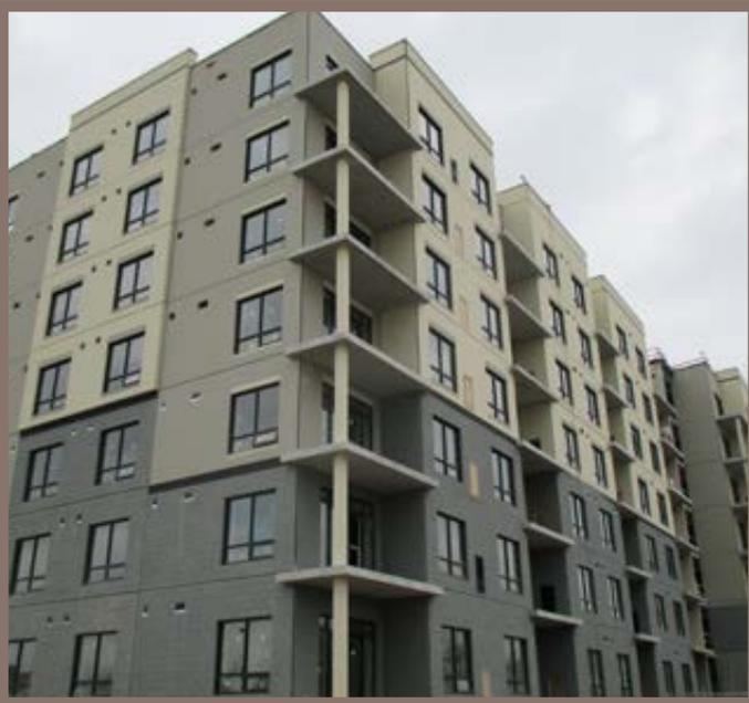
The Saginaw Garden building is a new 7 storey apartment building in Cambridge, Ontario, designed as a total precast structure. The majority of the structural components of the building are precast concrete. The apartment building includes 122 open-concept units with many amenities and condo-quality features, including large outdoor balconies. The building also features underground parking, a multi-purpose lounge and two large outdoor terraces.
