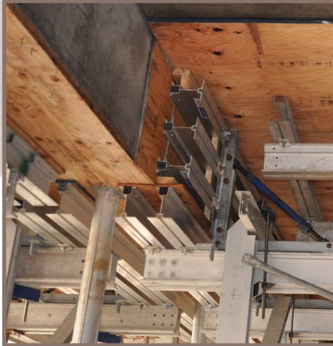
The 4-way sloped slab required the use of smaller tables (average 30 m<sup>2</sup> soffit area ranging from 6.5 m-11 m in length by 3.5 m in width tables), and each has a unique slab configuration that requires that table to stay at the same location on each subsequent level. A typical slab pour, approximately 375 m<sup>3</sup> of concrete and 1,200 m<sup>2</sup> of formwork, took 24 calendar days to complete a full cycle from one entire parking level to the next. At one point,
